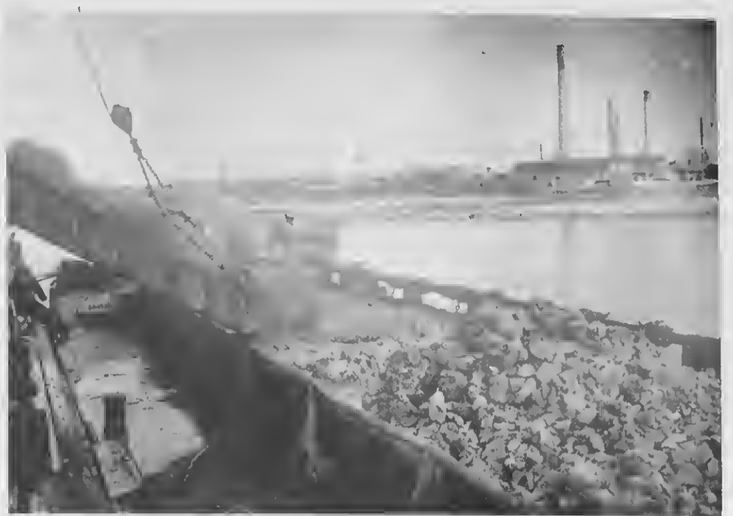
SPOIL is brought up from the bottom by the dredge's 44 buckets, dumped into the chute which sends it splattering into a barge. The barge is towed to sea where its load is dumped to a resting place hundreds of feet down.
